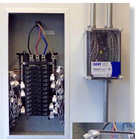
Right: The PowerScout is linepowered and the broadband power supply accommodates voltages from 80-600VAC. Left: The PowerScout 24 can use up to 24 CTs to measure any combination single or three-phase loads. Mix and match any of DENT's RoCoil or Split core CTs to monitor building mains and smaller loads simultaneously with a
