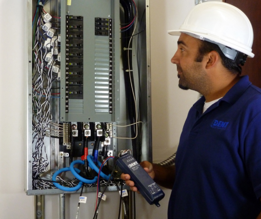
The Next Generation PowerScout 3 Plus with flexible Rogowski coils CTs minimize installation effort and cost.
