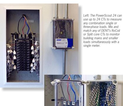
Right: The PowerScout is line powered and the broadband power supply accommodate voltages from 80-600VAC
